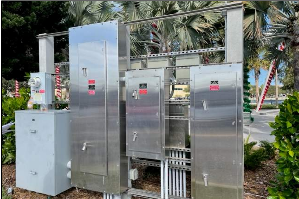
Photograph 41 – View of 208/120 V switchgear that will need to be re-fed in the South Basin.
