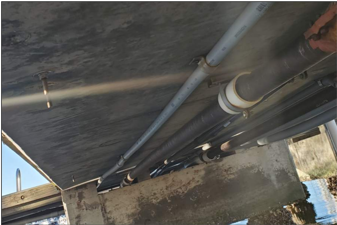
Photograph 37 – Existing fiberglass fuel piping below fuel dock in Central Basin.
