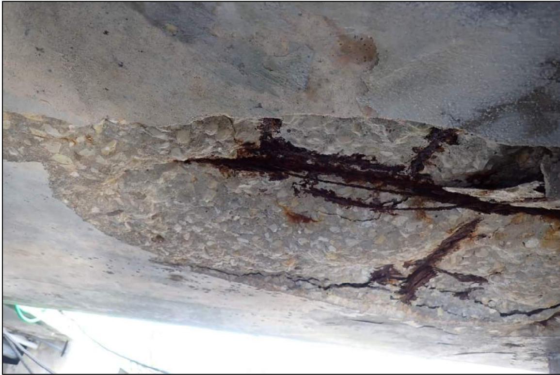
Photograph 3 – Typical open spalling with exposed prestressing strands on the underside of a South Basin finger pier deck slab.
