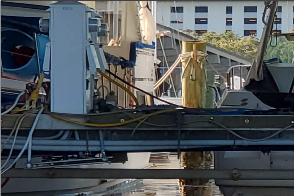
Photograph 35 – Existing comingled utility piping under piers at Central Basin.
