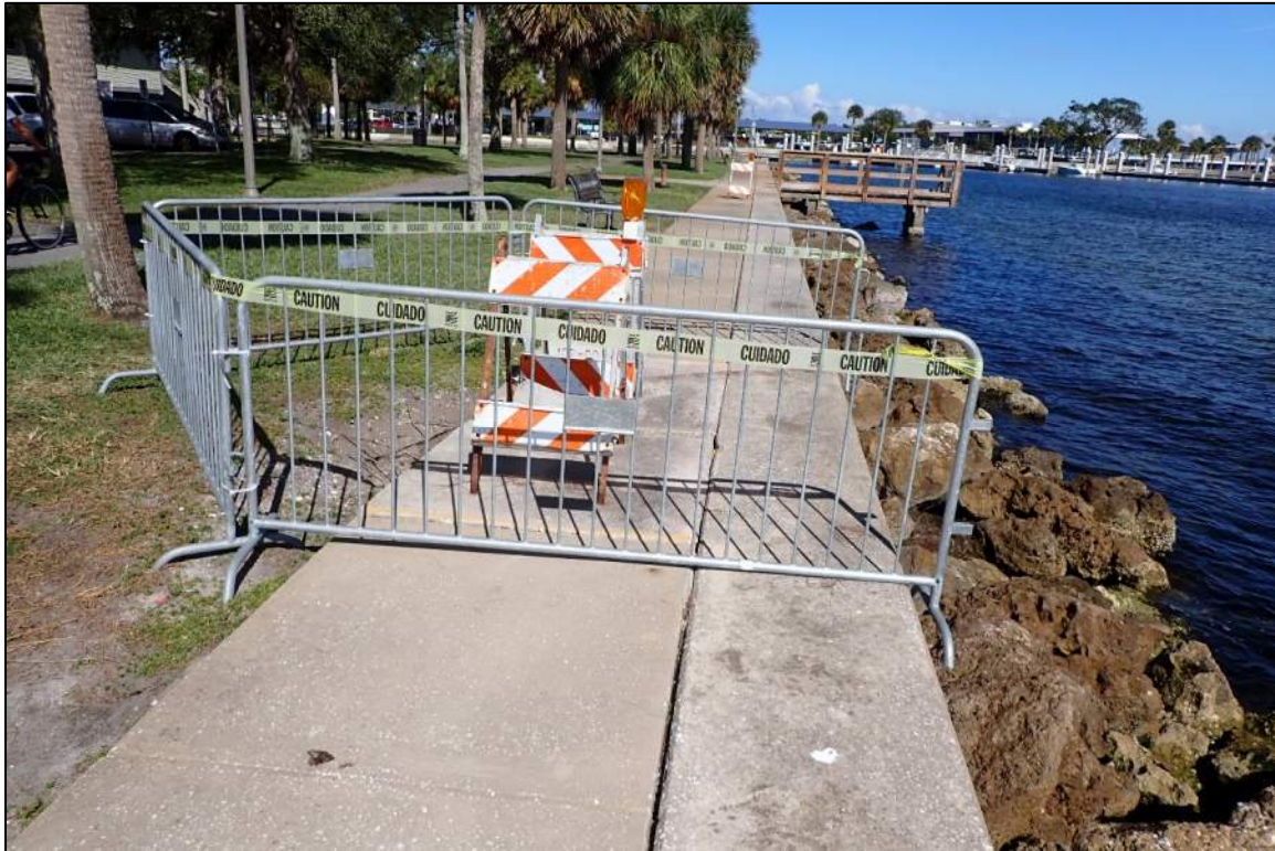
Photograph 7 –Sinkhole below walkway along eastern perimeter of Demens Landing.
