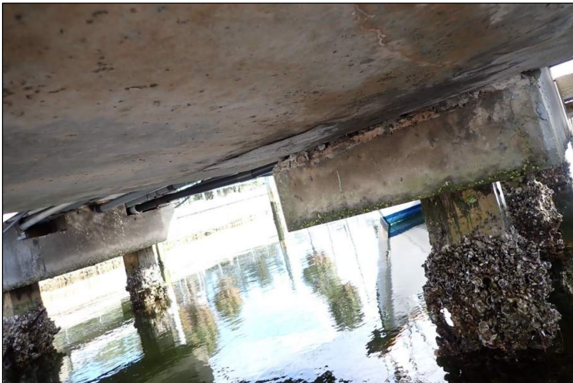
Photograph 8 – View of substructure in South Basin. Marine growth visible on piles and some cracking and deterioration visible on pile cap.
