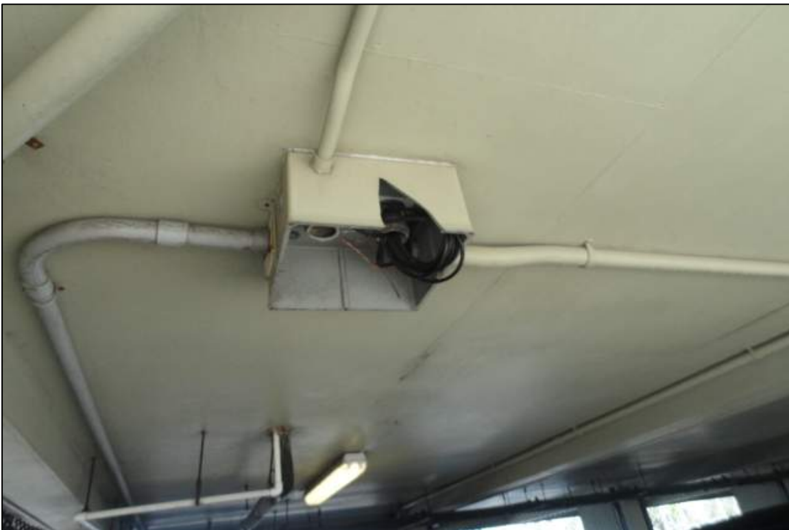
Photograph 26 – Marina Office and Ship Store, View of Damaged Electrical Junction Box at the Ceiling of the Open-Air Carport Ceiling.
