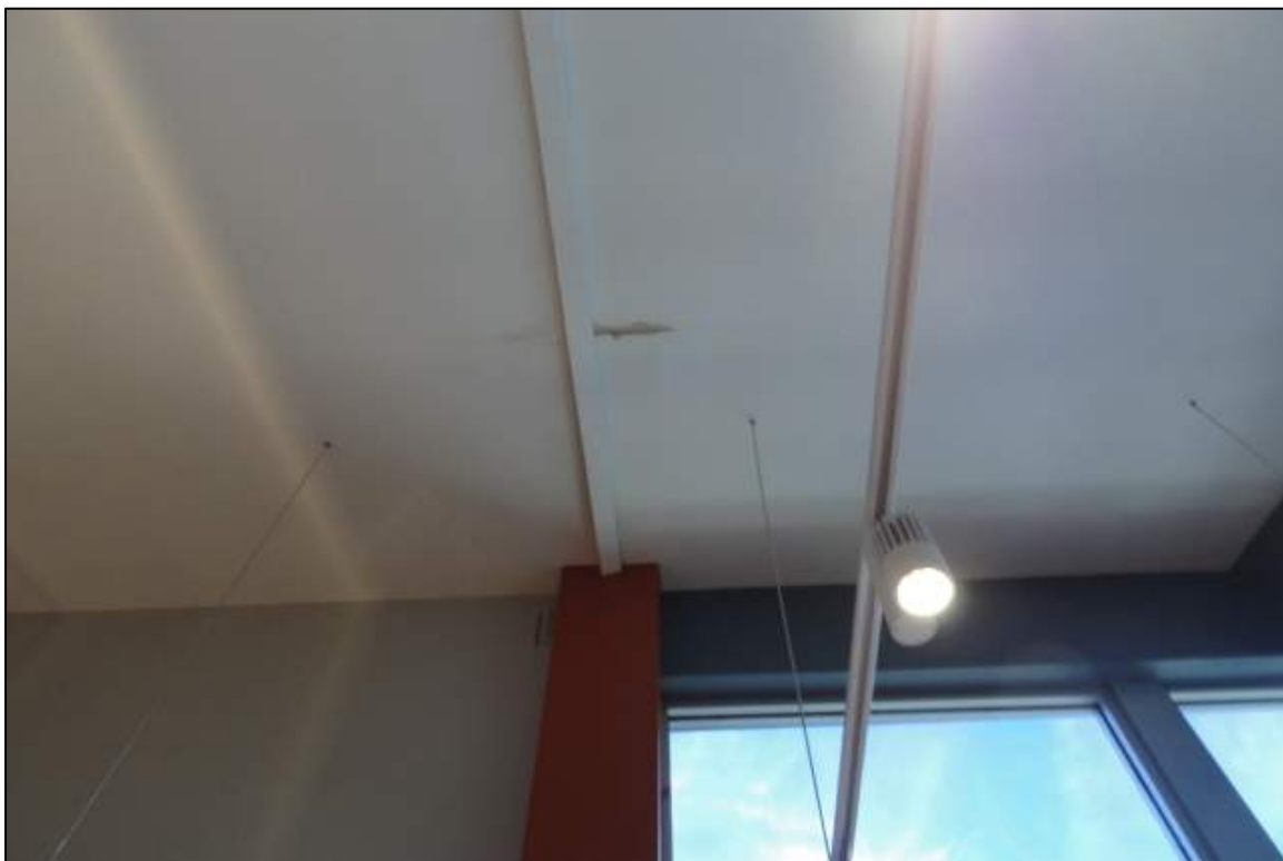
Photograph 28 – Marina Office and Ship Store, View of Damage to Local Area of Gypsum Board Ceiling due to Roof Leak.
