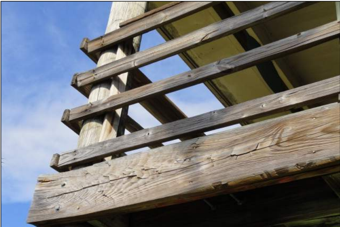
Photograph 12 – South Basin Comfort Center, View of Warped Timber Guardrails and Girder.
