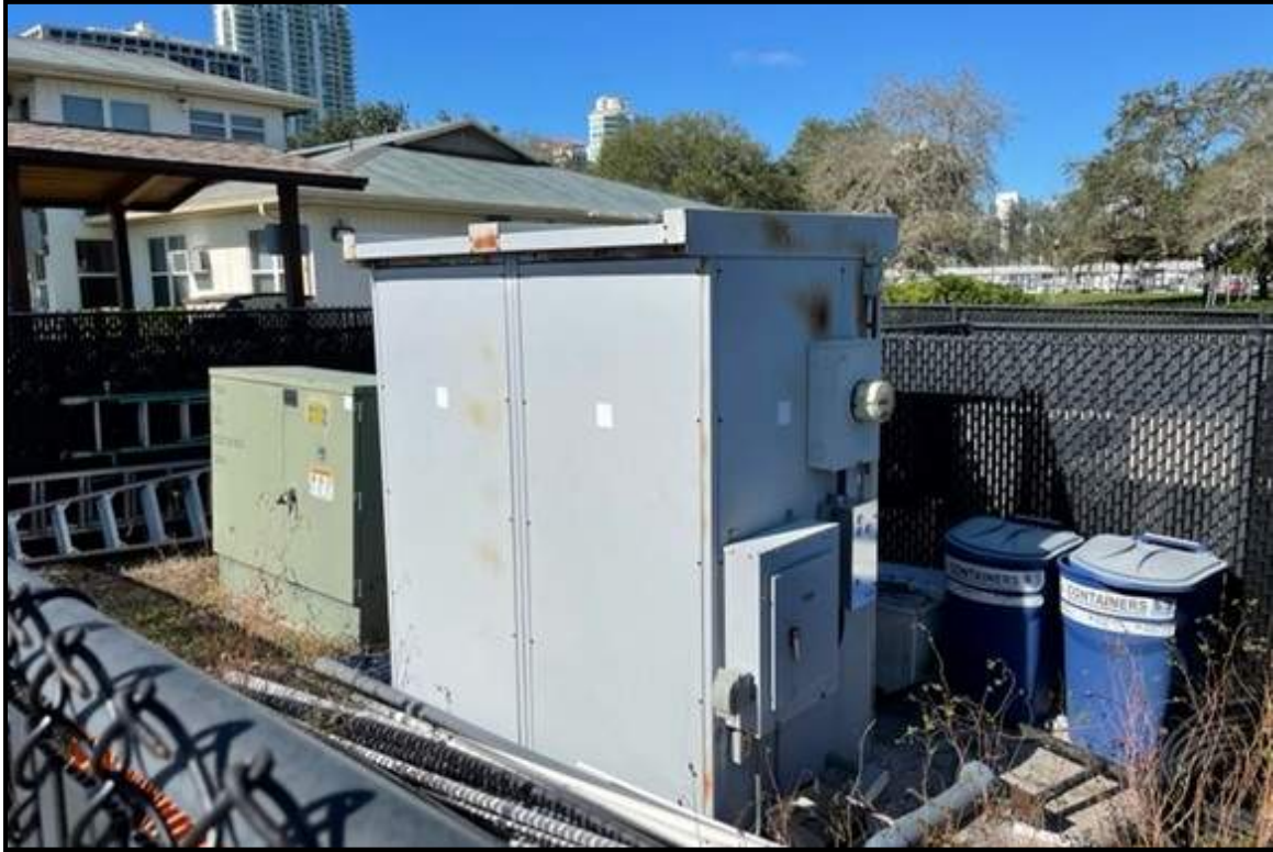
Photograph 40 – View of typical Duke Energy transformer and 208/120 V switchgear in the South Basin.
