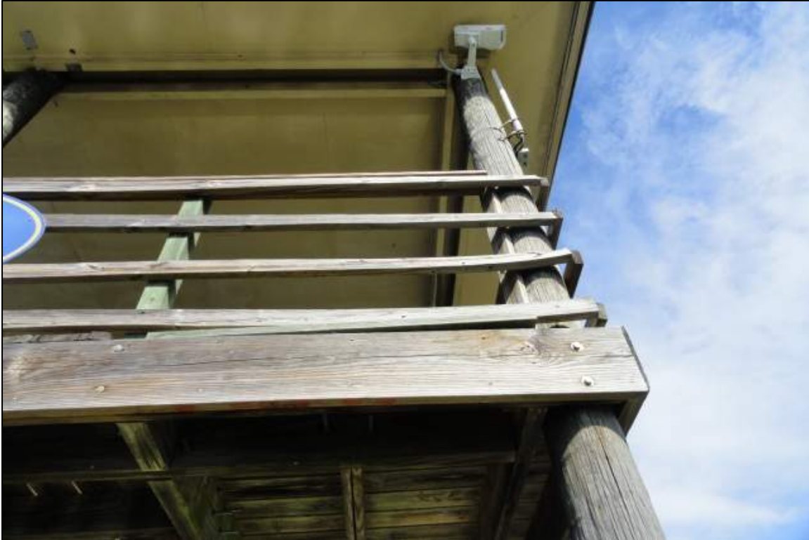
Photograph 13 – South Basin Comfort Center, View of Warped Timber Guardrails.
