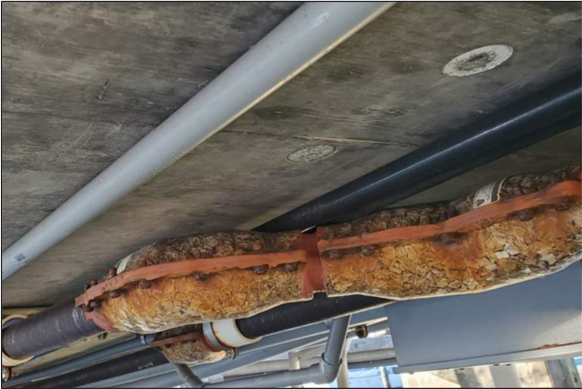
Photograph 38 – Existing clamshell sealed fitting fuel lines in Central Basin.
