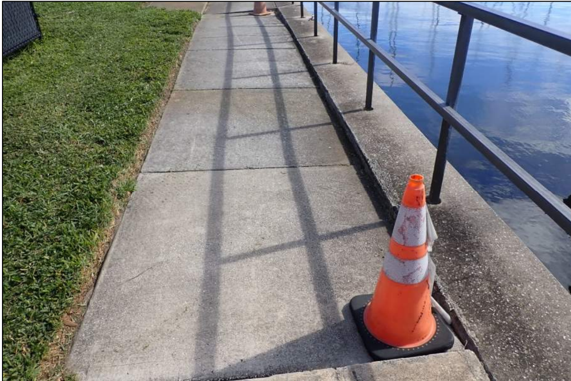
Photograph 6 –Deflection of walkway slab along South Basin seawall.
