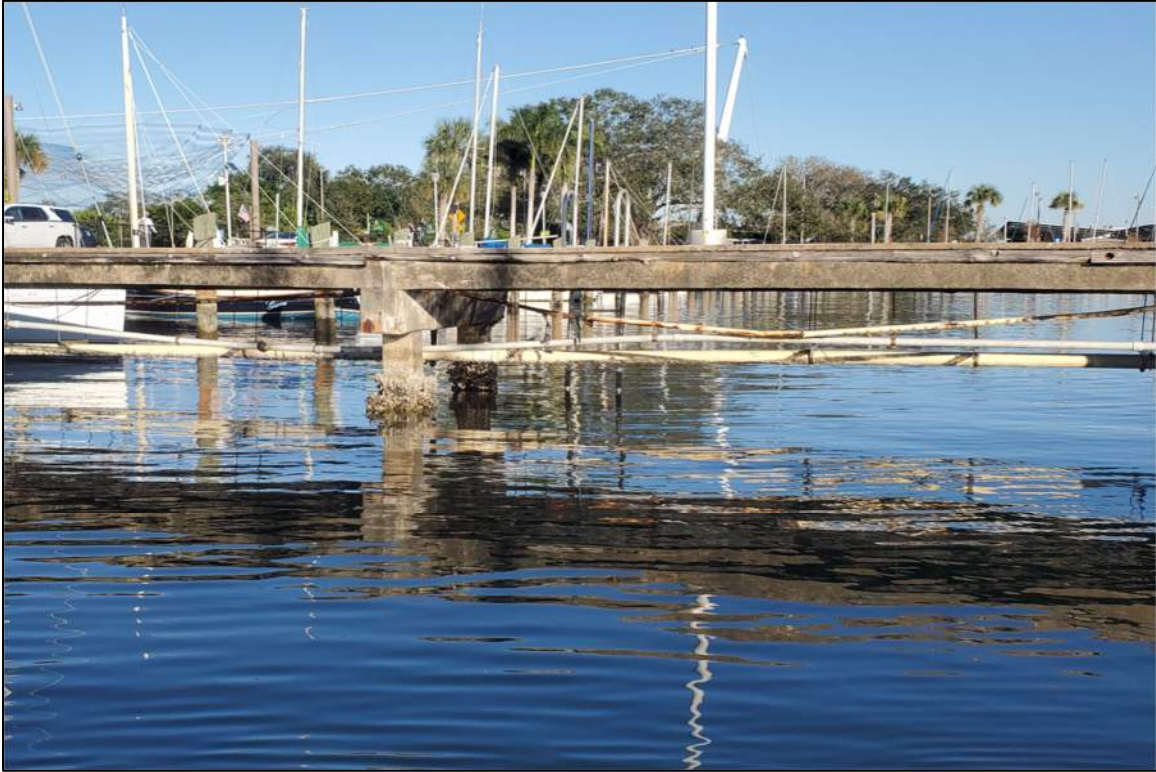
Photograph 34 – View of sagging utility (domestic water) lines at Central Basin.
