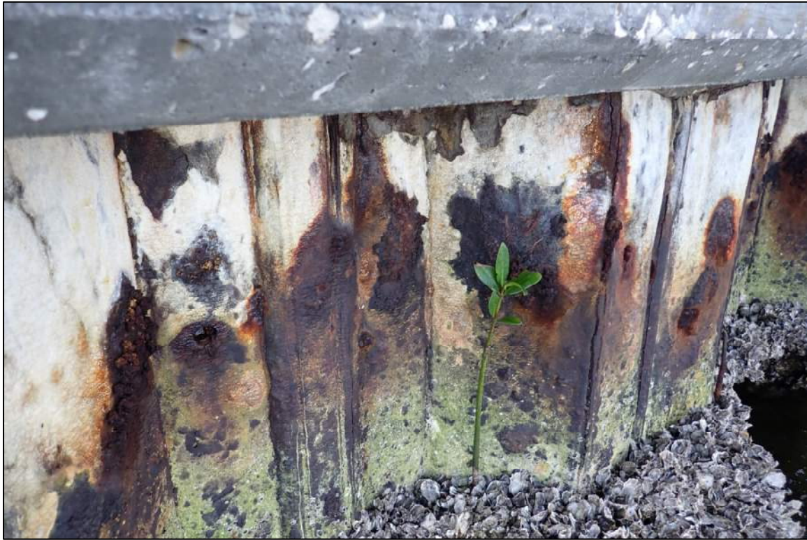
Photograph 5 – Typical condition of steel sheet pile bulkhead with widespread corrosion blistering and delamination at the knuckles.
